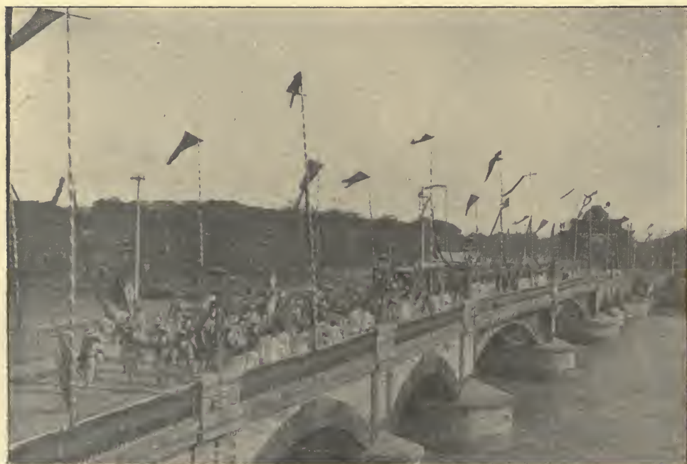
SPANISH REINFORCEMENTS CROSSING BRIDGE OVER PASIG RIVER.
